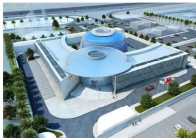
Traffic Management Center, Dubai
